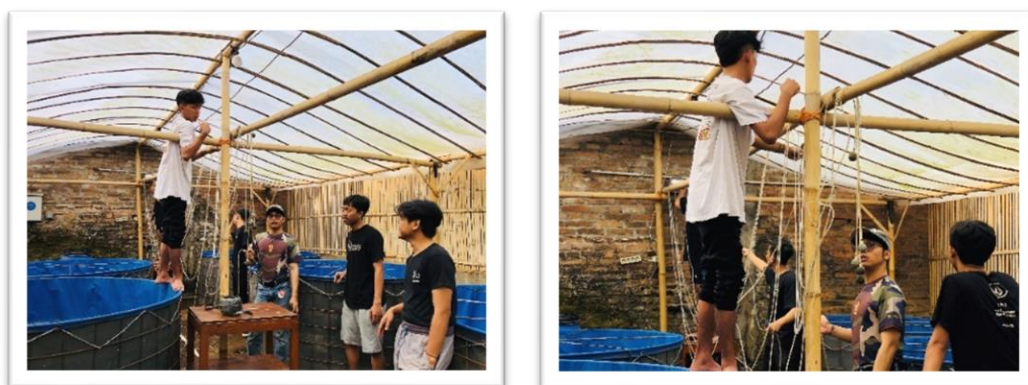
Figure 5. Aeration Hose Installation
